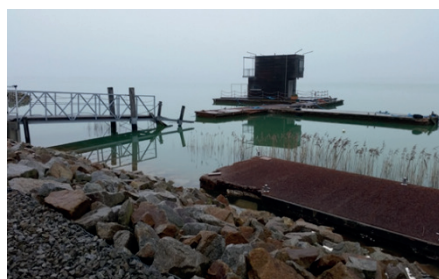
Fig. 2. A damaged accessway to the floating houses on Lake Partwitzer
