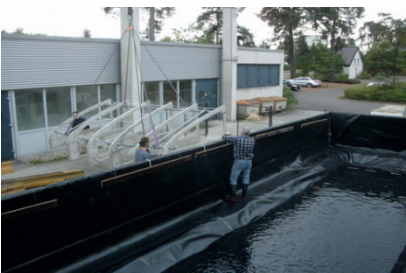
Fig. 8. Using the crane to lift the shock absorber
