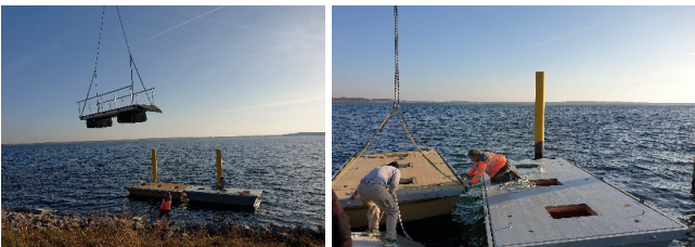
Fig. 7. The left photo: the assembly of the two pontoons; the right photo: using an assembly crane to make an accessway
