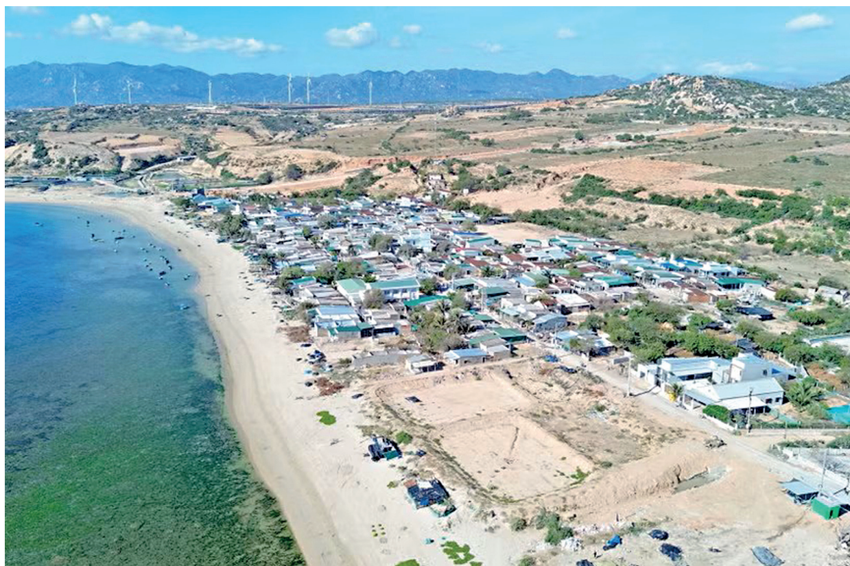
Fig. 2. Construction site of the Ninh Thuan-1 NPP
