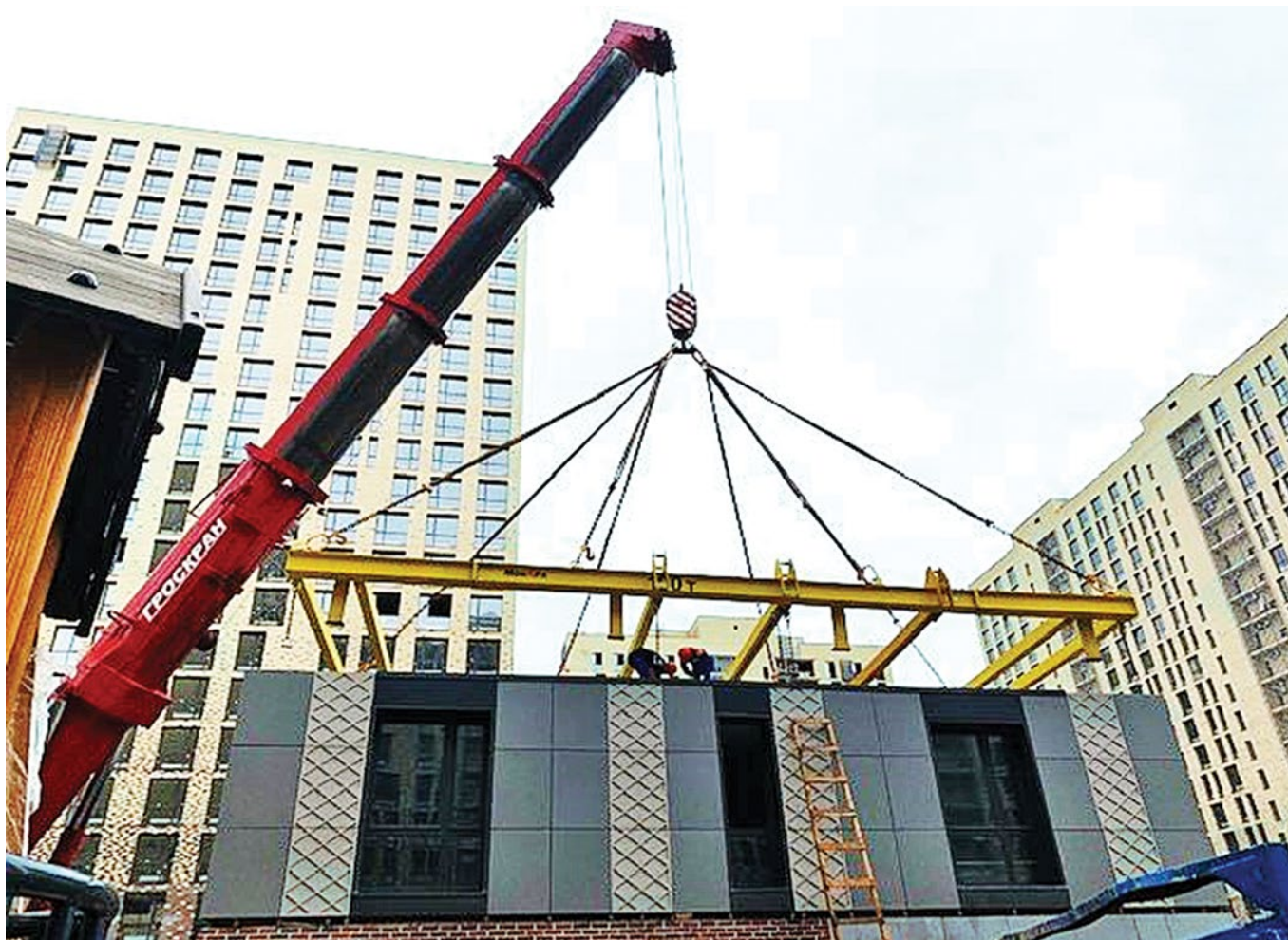
Installation of a large-sized volumetric block (a module)
