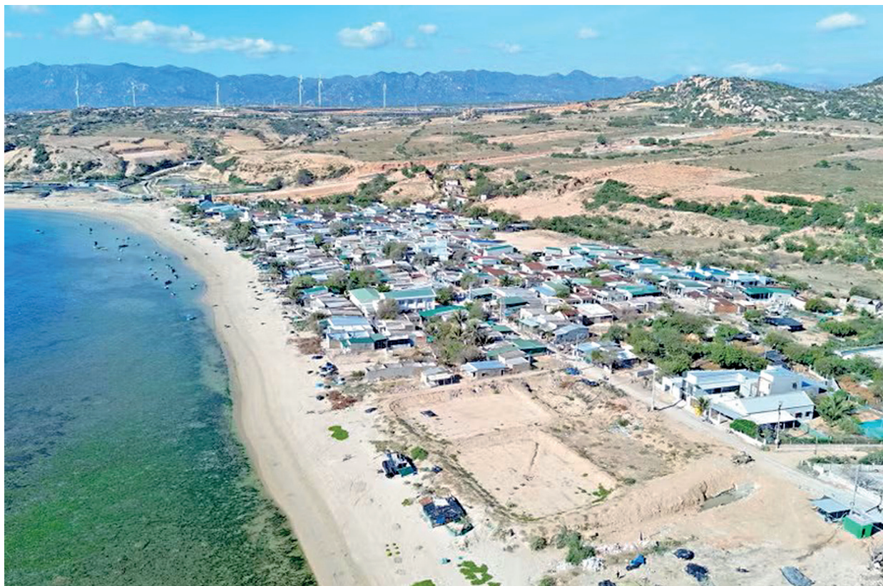
Fig. 2. Construction site of the Ninh Thuan-1 NPP
