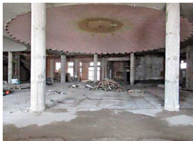
Fig. 5. The general view of the first-floor premises
