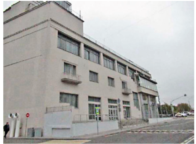
Fig. 1. The building facade fragment
