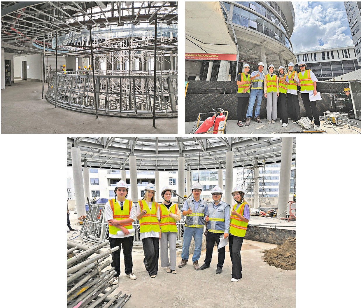
Fig. 8. Work on the construction site of the facility “VAN LANG University”
