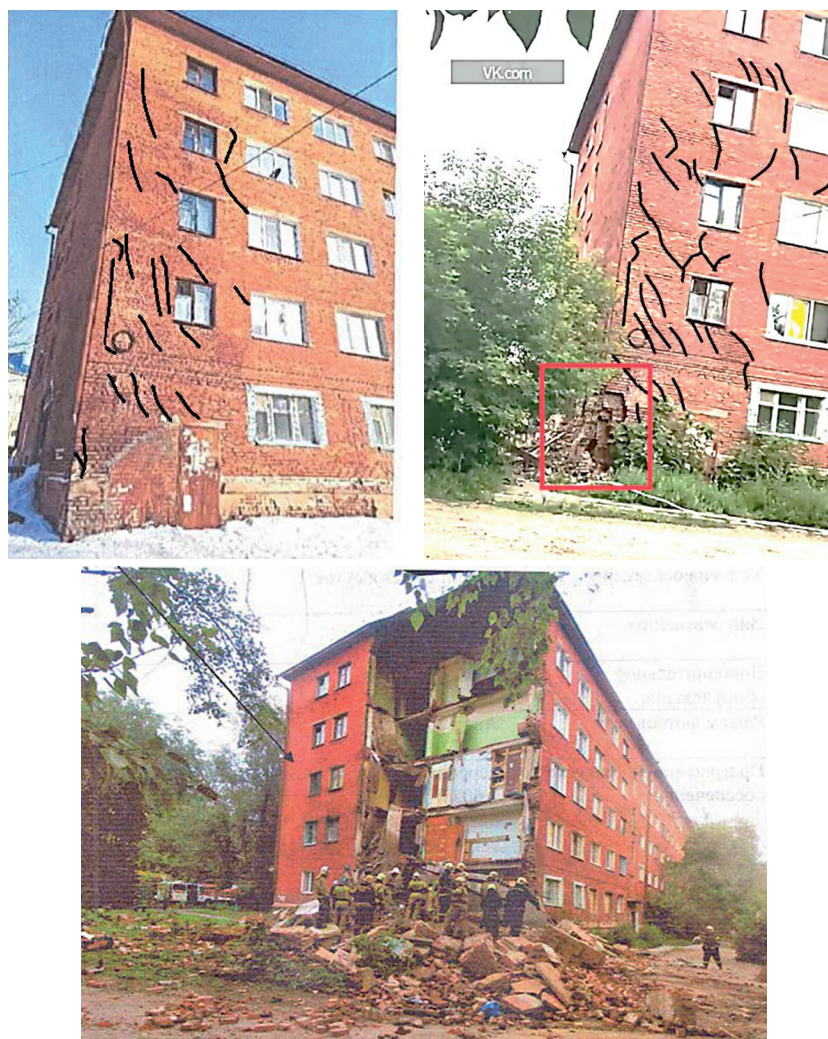
Fig. 4. General view of an apartment building in XX Partsezda St. in Omsk before and after the collapse (the arrow shows the progressive destruction of the corner section of the outer wall a few seconds before the collapse of the end part of the building)
