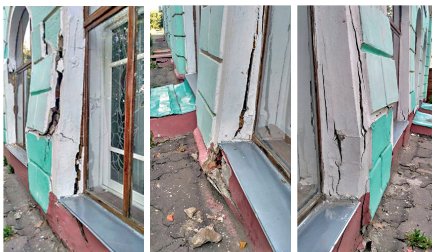
Fig. 3. General view of an apartment building along the Dubrovinsky Embankment in the city of Orel after the collapse: a — emergency condition of the first-floor walls; b — recorded before the collapse
