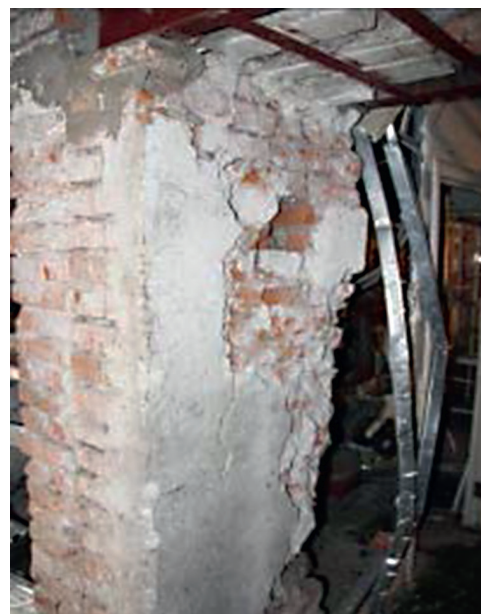
Fig. 2. View of the pillar of the non-designed opening in the basement, which was the source for activating the process of destruction of the building (the state of the pillar, recorded before the collapse of the corner of the building)
