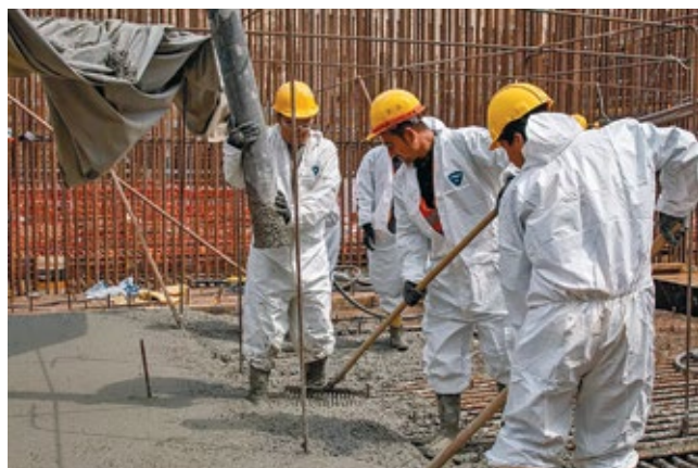
Fig. 4. Concreting process of turbine unit foundation
