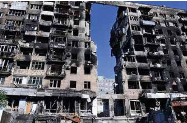
Fig. 3. The destruction of an apartment building that cannot be restored
