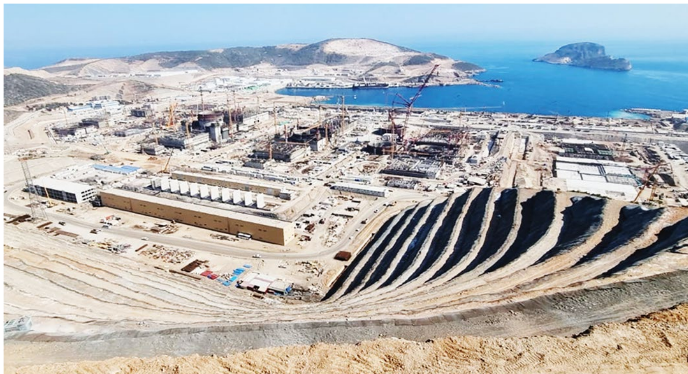
Fig. 2. NPP Akkuyu construction site, Turkey, 2022
